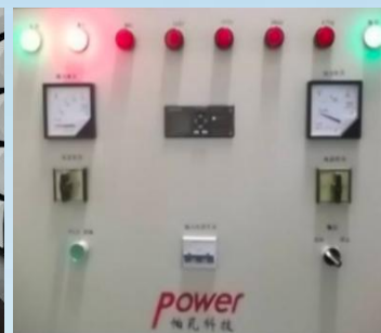
Finished Product Wide Voltage Impulse Test
